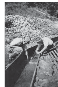
Searching for Gold in a Sluice Frame
